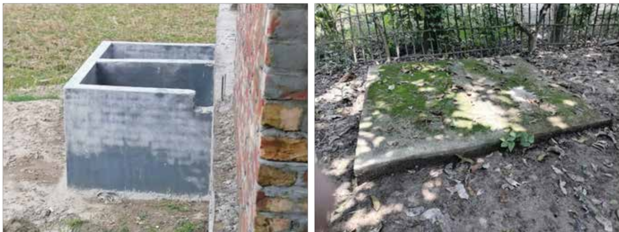
Figure 4: Septic Tank and Fully Lined Tank in Muktinagar
