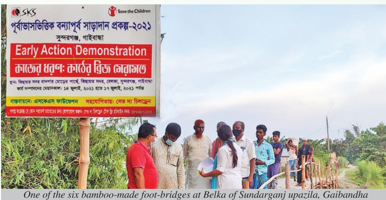
One of the six bamboo-made foot-bridges at Belka of Sundarganj upazila, Gaibandha
